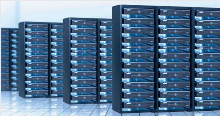
VODAFONE BUCCINASCIO 2015 Buccinasco (Italy) Application: Data Center Plant type: Hydronic System
